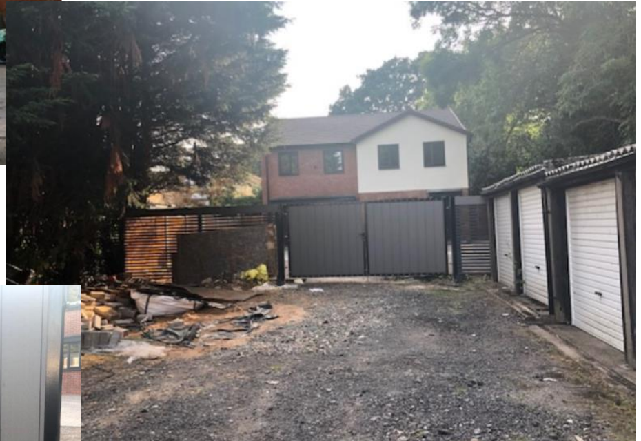
Fence and gates to the front of properties
